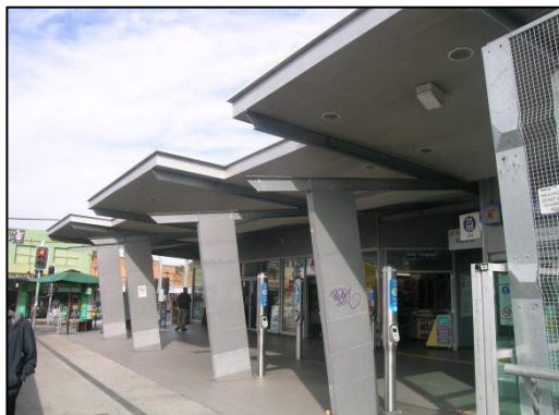
Photograph 19: Riverwood Railway Station, looking southwest from Belmore Road.
