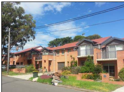
Photograph 7: Example of multi dwelling housing fronting Lawrence Street.
