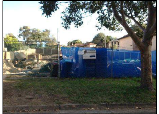
Photograph 12: Property under construction at No. 31 Lawrence Street.
