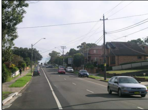
Photograph 21: Bonds Road, looking north.
