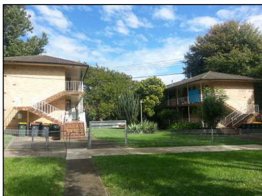
Photograph 9: Two (2) storey residential flat building fronting Jaques Avenue.
