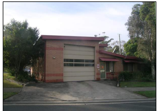
Photograph 18: Peakhurst Fire Station fronting Jacques Avenue.
