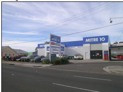
Photograph 25: Mitre 10, on the south side of Forest Road.
