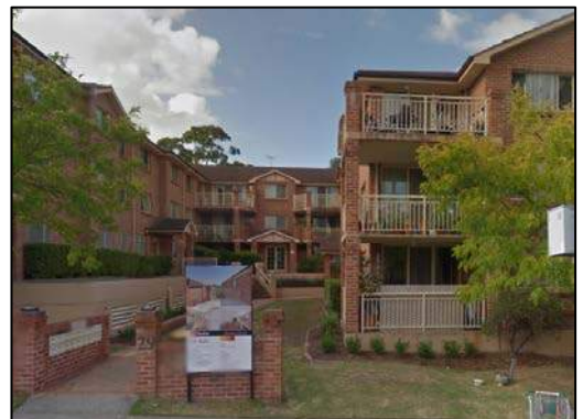
Photograph 20: Example of a three (3) storey residential flat building fronting Littleton Street.
