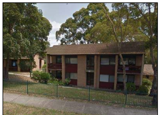
Photograph 10: Two (2) storey residential flat building fronting Bonds Road.
