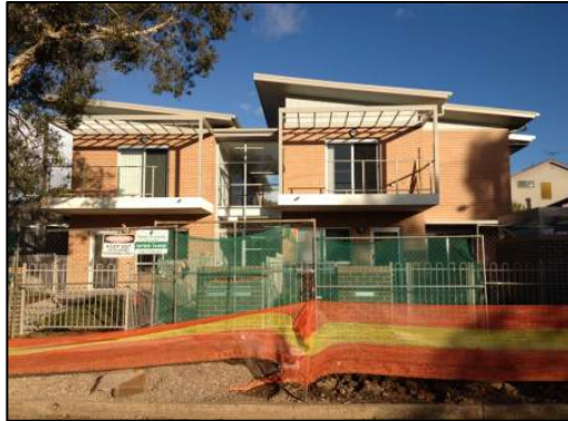
Photograph 11: Two (2) storey residential flat building under construction at No. 1 Gover Street.
