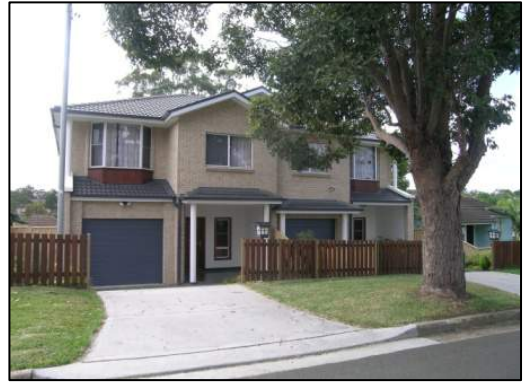
Photograph 6: Contemporary semi-detached dwellings fronting Gover Street.
