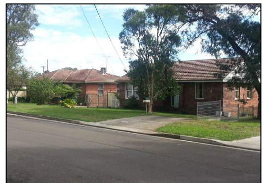
Photograph 4: Example of dwelling houses fronting Richards Avenue.
